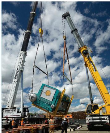
regulations. Specialized logistics planning and a custom heavy-haul trailer ensured a safe journey to the customer site. Upon arrival, two high-capacity cranes were used to rotate the boiler to its upright position and place it precisely onto its final foundation. The entire delivery and rigging process was carefully orchestrated and smoothly executed, reflecting the expertise of both Nationwide Boiler's project team and our trusted partners.
